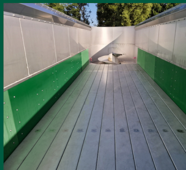
Surfaces in contact with substrate made of stainless steel or with plastic cladding.
